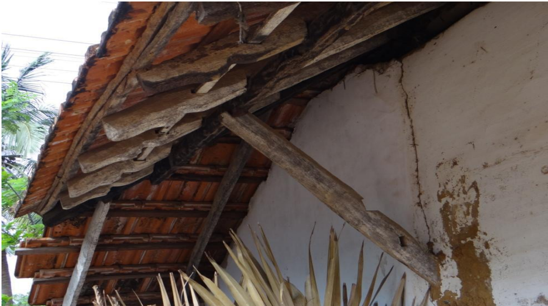
Details of Traditional House in Kumbharam Village
