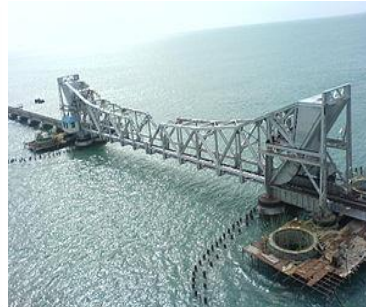
Re-engineering Pamban railway
